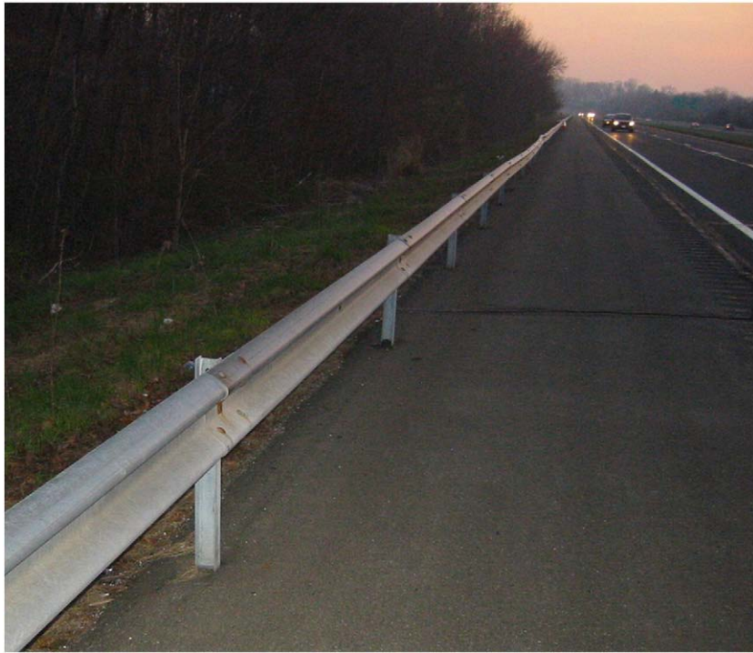
Fig. 1. W-Beam Guardrail along Interstate 87, New York State.
