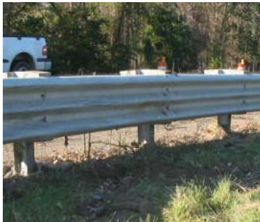
Figure 4 – Strong Post Thrie-Beam Barrier (NASS/CDS Case 2007-011-152)
