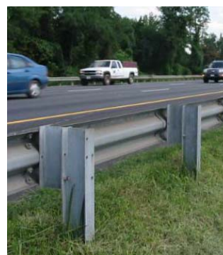
Figure 2 – Strong Post W-Beam Barrier (NASS/CDS Case 2003-009-167)
