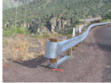
Figure 7 – Guardrail End Terminal (NASS/CDS Case 2006-076-065)
