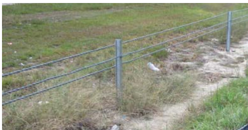
Figure 6 – Cable Barrier (NASS/CDS Case 2007-043-166)
